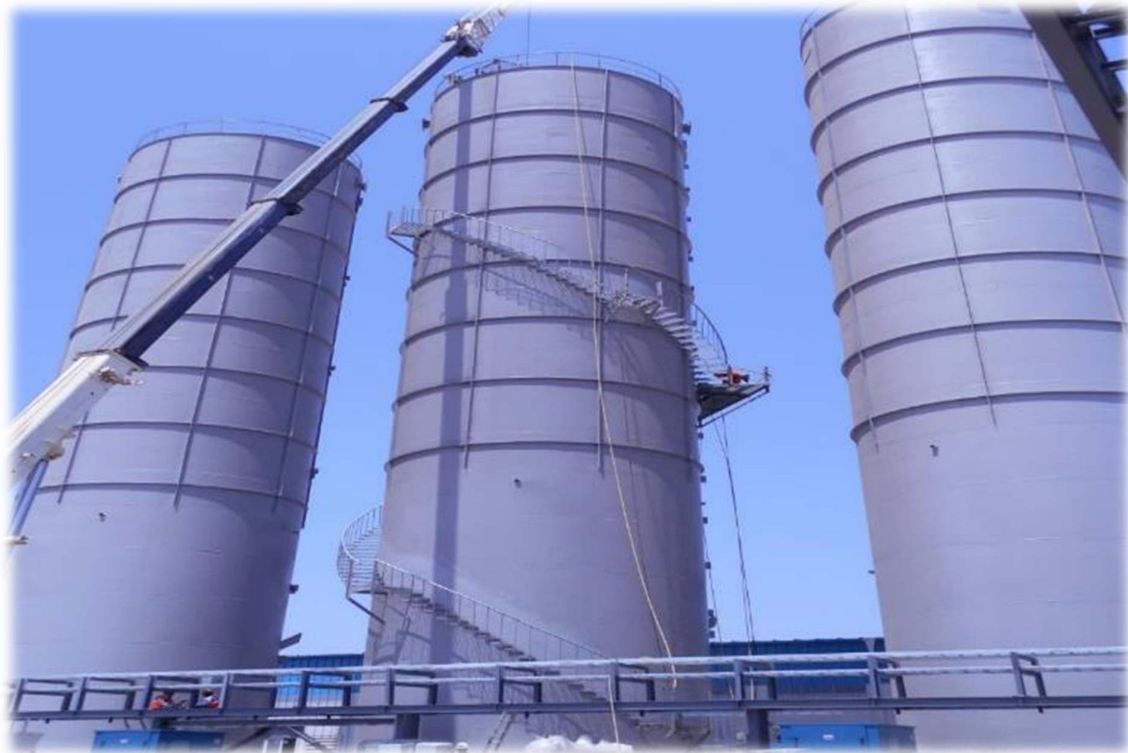
Design, Fabrication, supply & Installation of Silos at Lubrizol (Dahej)
